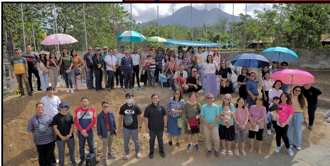
With the Mt Makiling on the background, Single Working YPs and Young Couples from Lighthouse BBC Tatalon, Cainta, Pasig and Taguig, along with Pastor Reuben, Pastors and Pastor's Men pose for a picture at the site of the Lighthouse Cafe being constructed at the Lighthouse Manifold Grace Center in Sto Tomas, Batangas.
